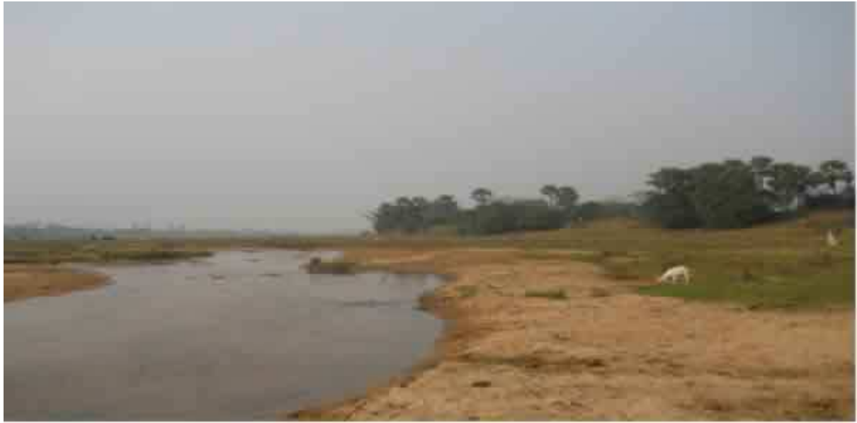
Fig. 2.14: Indisposed bed of River Chandan due to excess excavation of sand.
